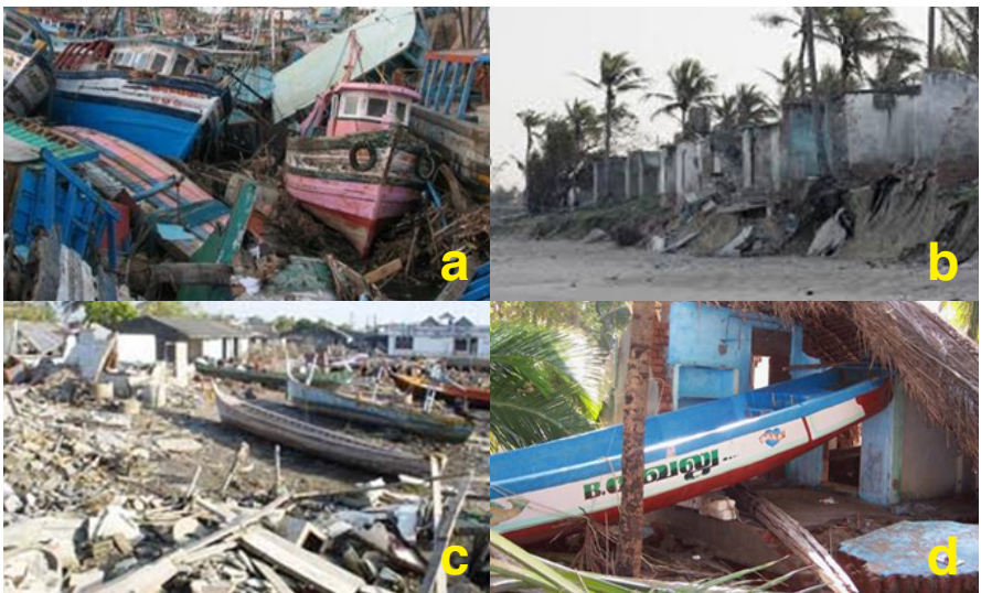
(a) Tsunami damages in Cudalore; (b) Erosion in Pondicherry; (c) Houses damaged in Nagapatnam; (d) Boats damaged in Cudalore
