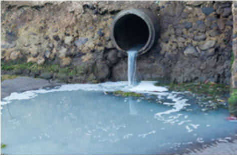
Figure 2C. Sewer outfall, Station 3. Note: foamy, bluish and whitish effluent. 8-26-2022
