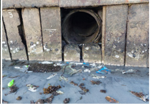
Figure 2B. Sewer outfall south of Station 2 12-15-2023
