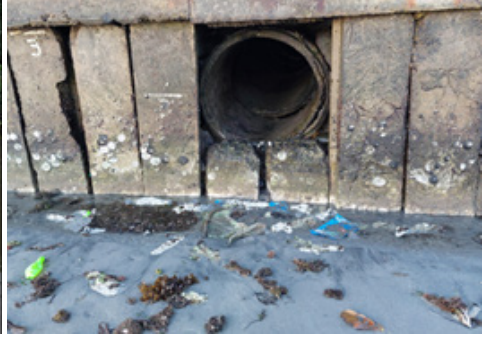
Figure 2B. Sewer outfall south of Station 2 12-15-2023
